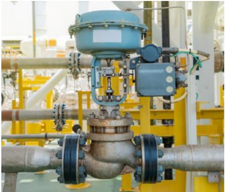
Figure 1. Actuated control valve
